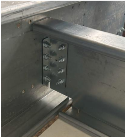
Fig 2. Bolted connection of profiles. Fig 3. Fragment of a connecting plate.
